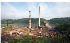
Brandenburg was contracted to demolish an operating zinc smelting facility and refinery in a ten month time frame. Built in the early 1930's, the site occupied on over 300 hundred acres and included more than 80 buildings. The main plant area was fully operational during the first three months of demolition. Buildings included one-story offices, six-story manufacturing facilities, and a seven-story power plant with a height exceeding 100 feet.
